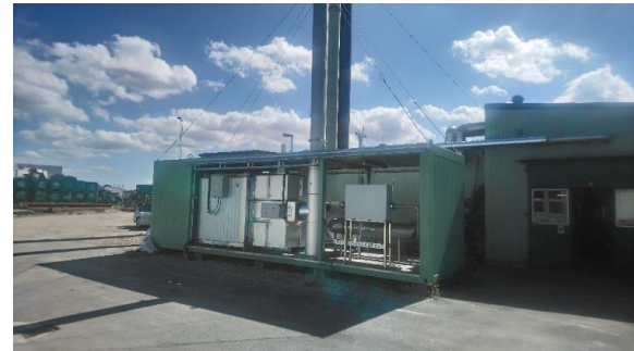
Figure 2. The fully containerized FRTO unit for low calorific LFG, commissioned August 2018 in Visby, Sweden.
