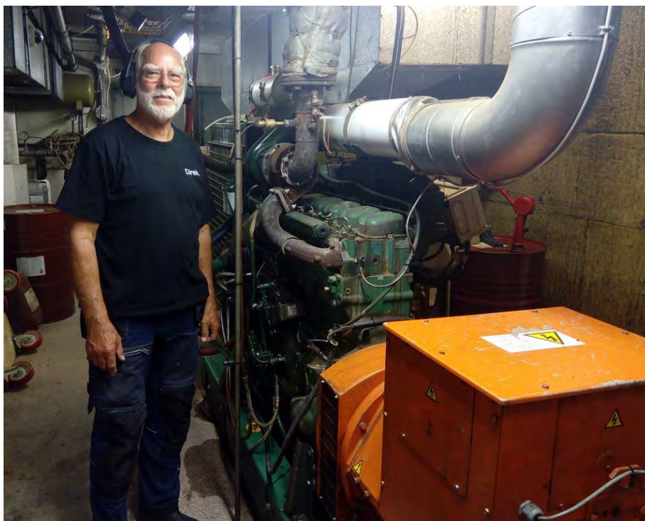
Figure 5. Ole Elmose, Managing Director Deponigas ApS besides a Volvo Penta engine modified to operate in dual fuel mode at Hedeland, Denmark.
